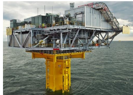
Figure 12 An example of an offshore substation platform on monopile foundation, Triton Knoll Offshore Wind Farm (RWE).
